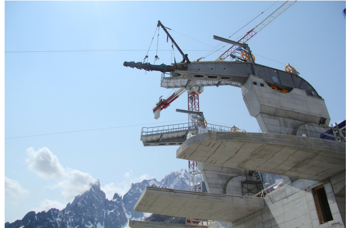
Building yard of the top station
