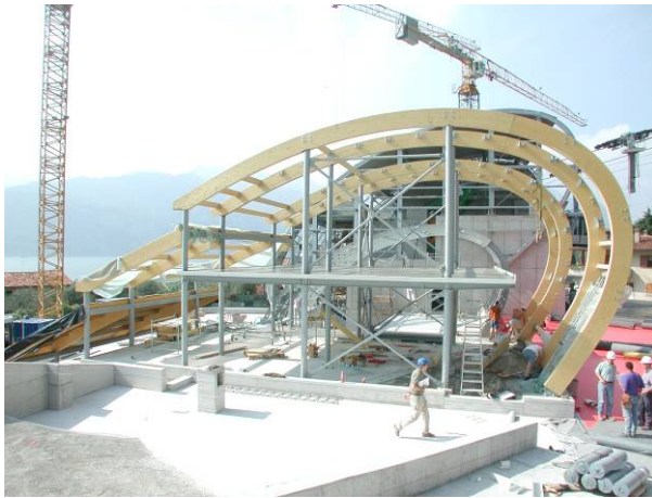
Building yard of the bottom station
