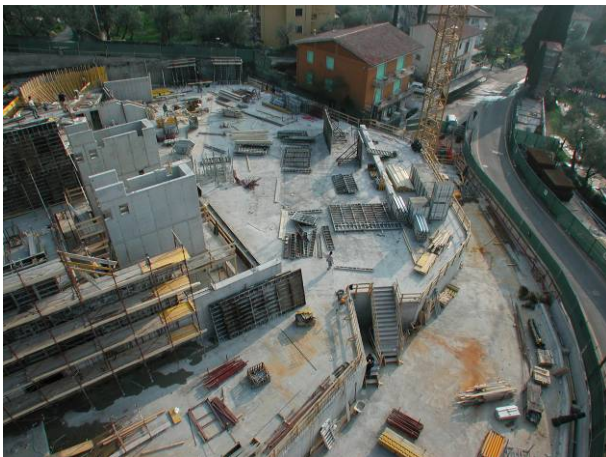
Shifting of existing road and underground parking
