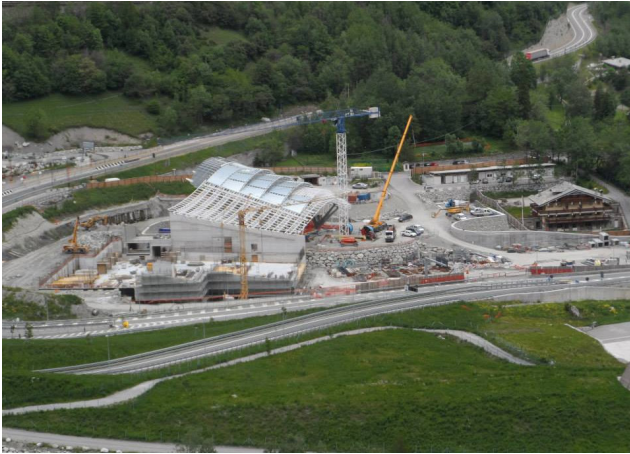
Building yard of the lower station
