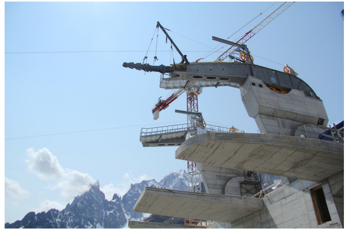
Building yard of the top station
