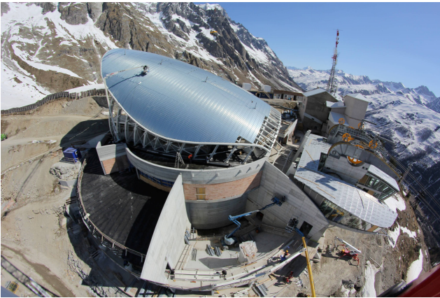
Building yard of the lower station
