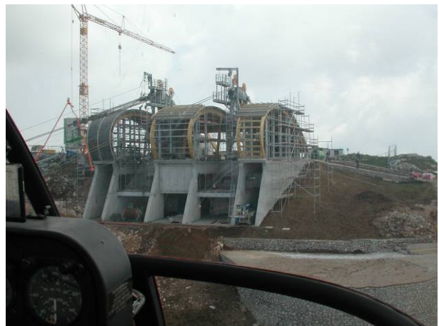
Building yard of the top station
