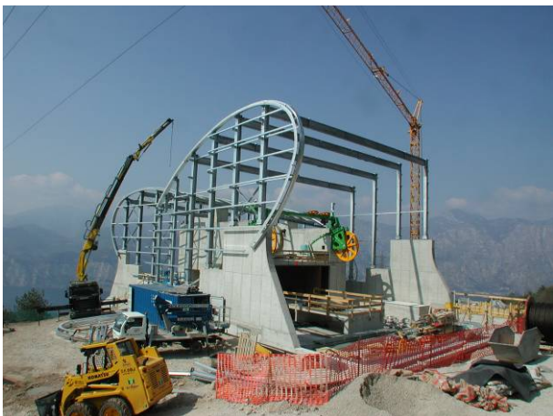
Building yard of the middle station
